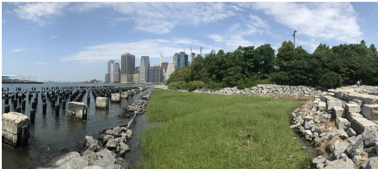
Figure 4-18: Rock Sill and Wetland as NNBF in Brooklyn Bridge Park, Brooklyn, NY
