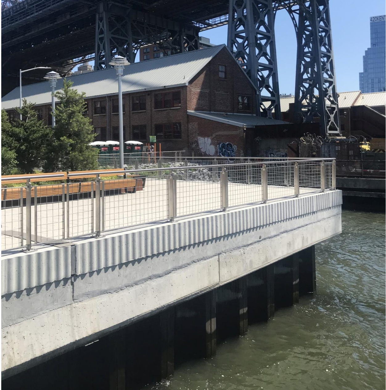
Figure 4-8: Bulkhead at South 5 th Street Brooklyn, NY
