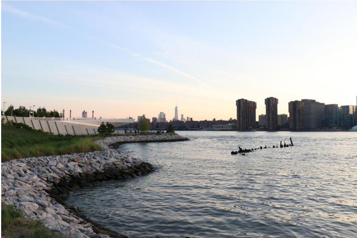
Figure 4-13: Revetment Hunters Point, NY (photo credit: Nicole Avella)
